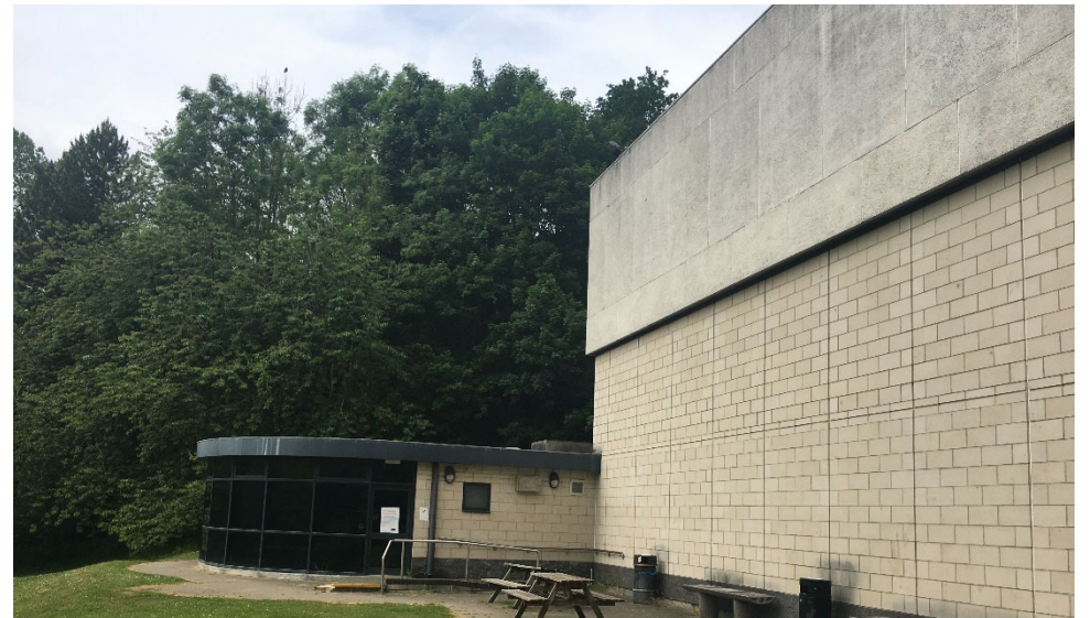
Southern elevation of the DLI overlooking the landscaped grounds
